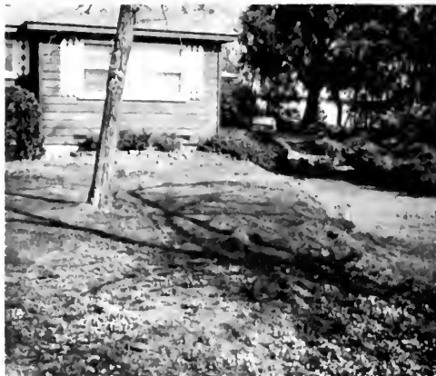
Photo 4. Undamaged wood-frame home on Foothill Boulevard in Sylmar fault zone. East view. Edge of thrust zone runs a few feet from the house across the lawn.
